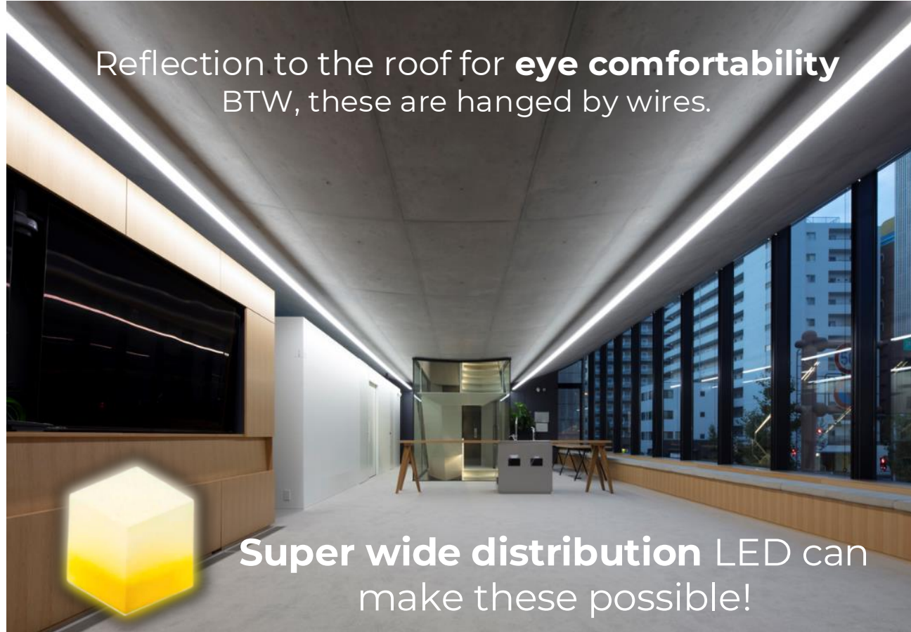
Takenaka Shizuoka sales office, Shizuoka city
