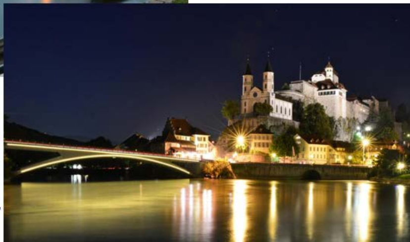
Maillart Bridge - Aarburg, Switzerland
