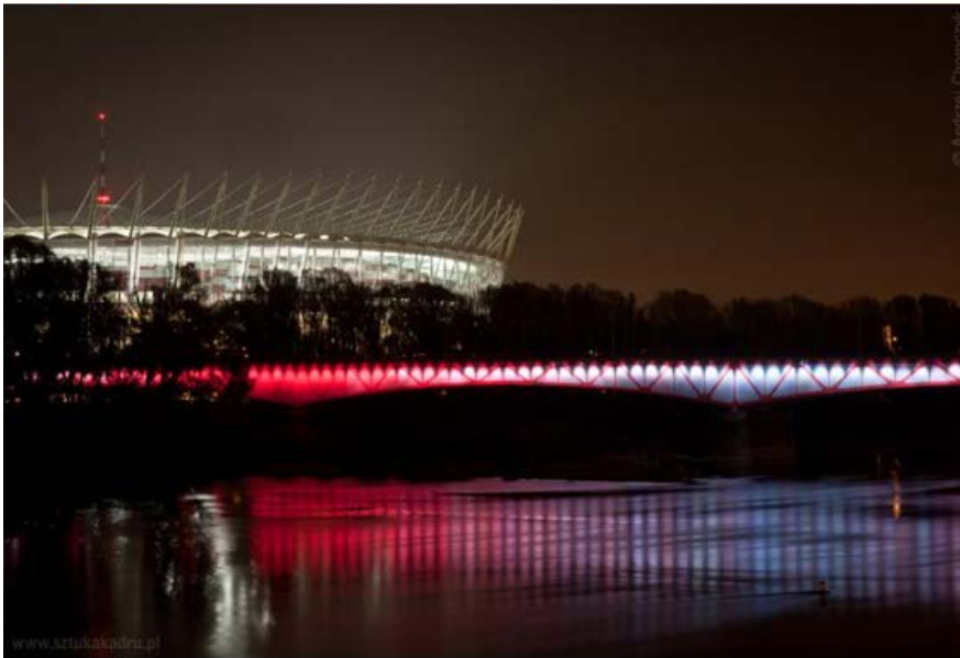
Railway Bridge – Warsaw, Poland
