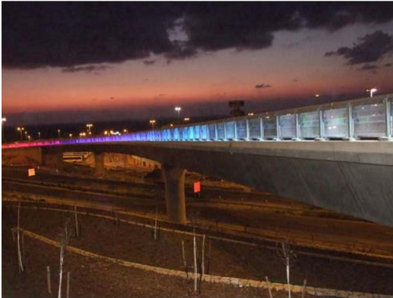
Haifa Bridge - Haifa, Israel Architect : Lighting centre
